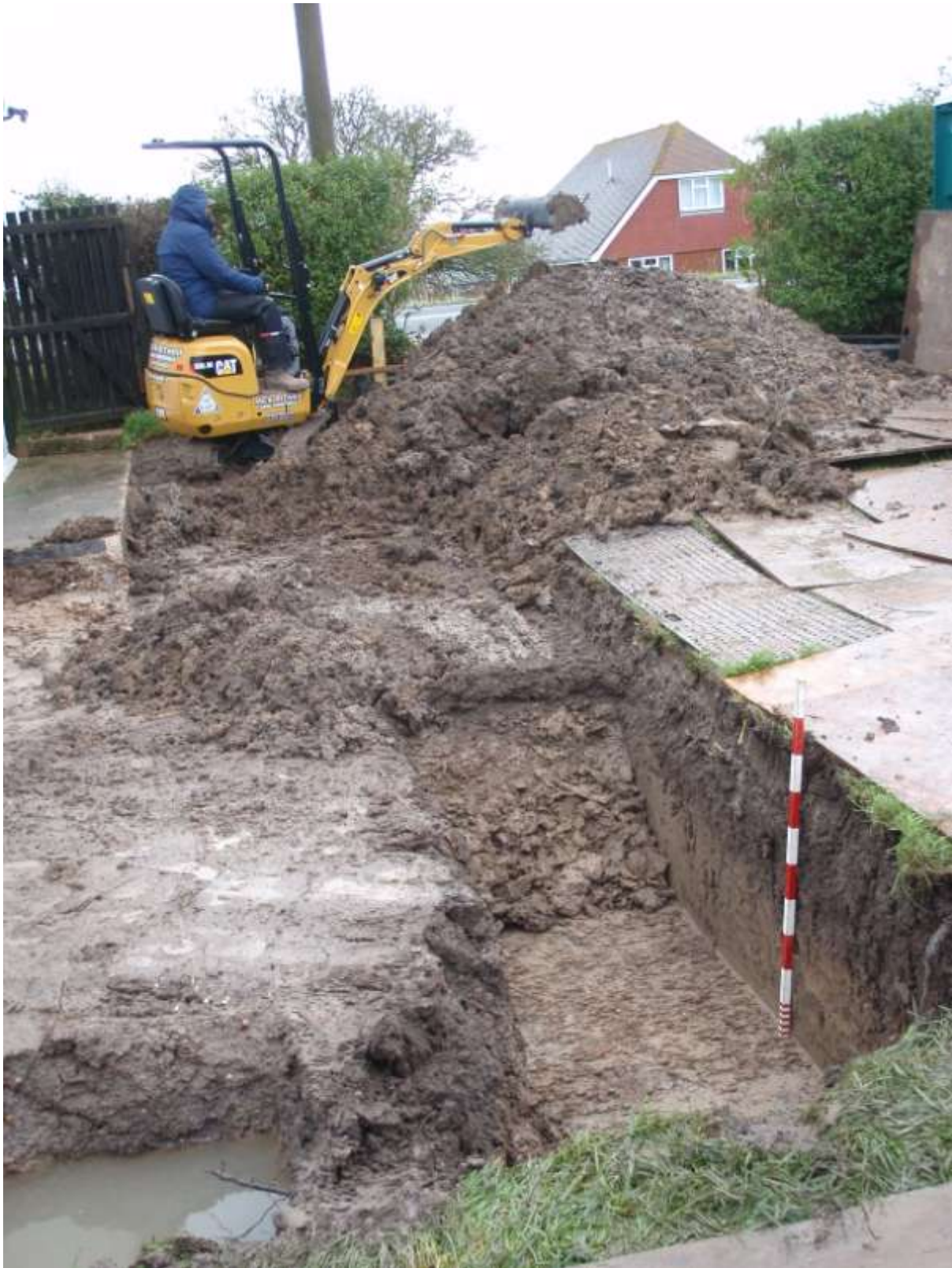
Plate 4. The site showing cutting of foundation trenches on the east side
