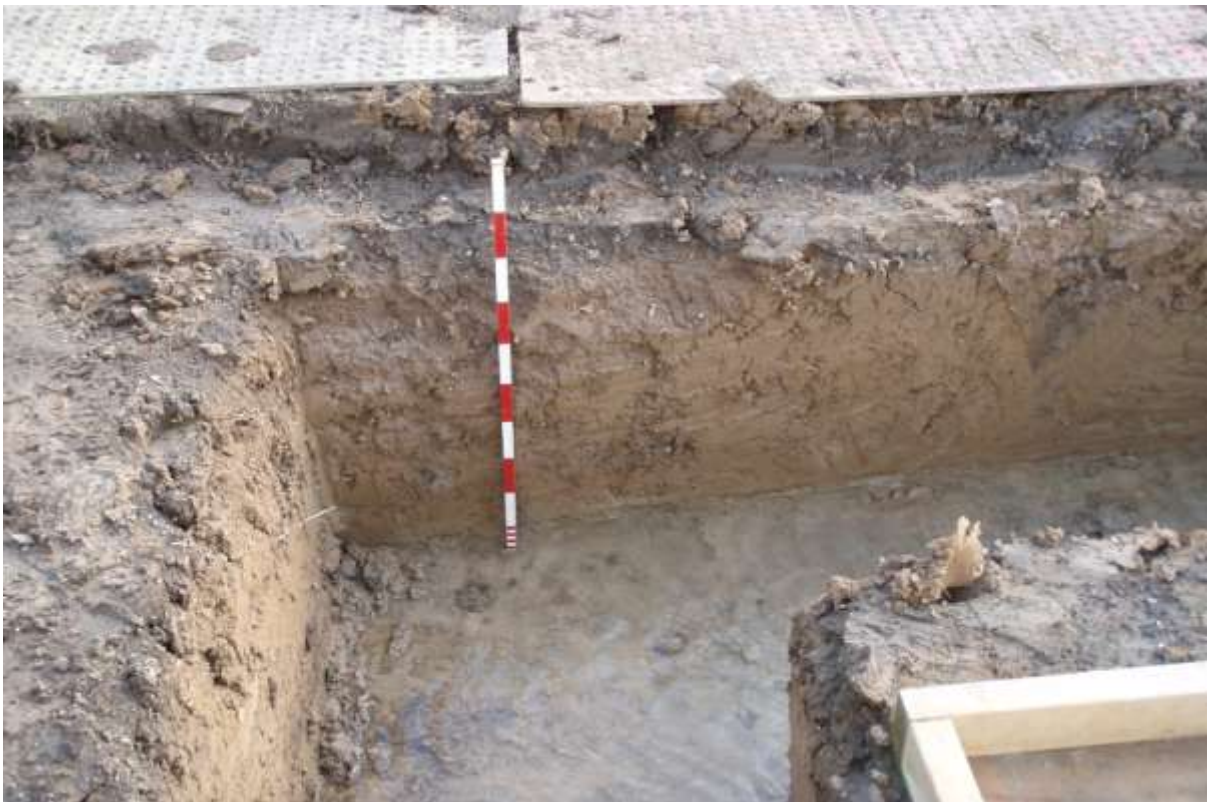
Plate 9. Completed foundation trenches on the south side
