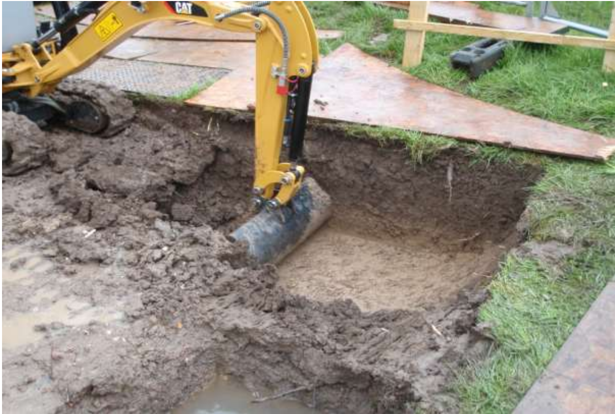
Plate 5. Digging foundation trenches on the east side
